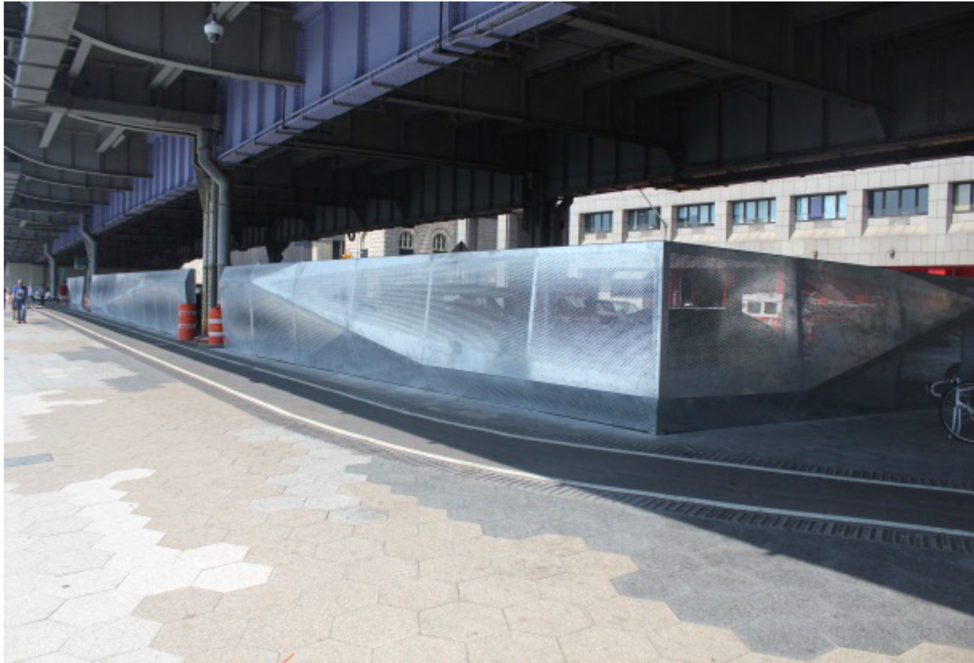
Finished project covers parking lot for FDNY
